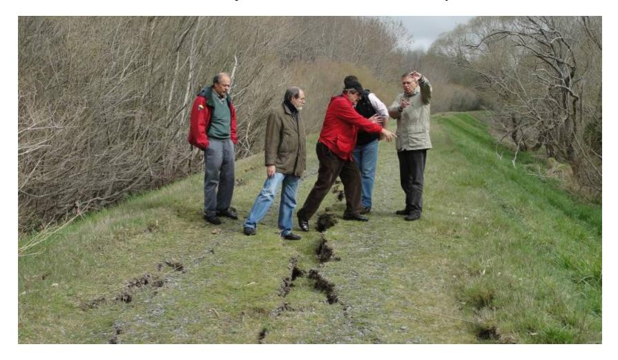
Failure of embankment of Waimakariri river due to lateral spreading. Liquefaction affected its environment. The river is just at the right side of photo.
