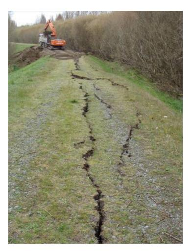
Failure of embankment of Waimakariri river due to lateral spreading. Liquefaction affected its environment. The river is just at the left side of photo.
