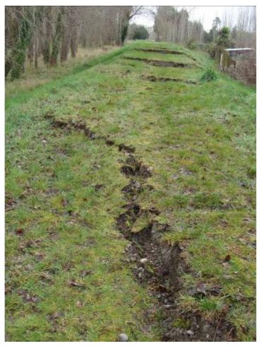
Failure of embankment of Waimakariri river due to liquefaction of its surroundings. Lateral spreading assisted The river is just at the left side of photo.
